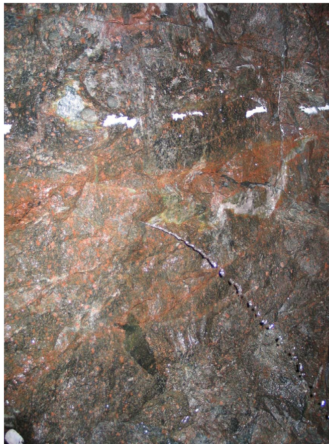
Figure 2-1. Tass-tunnel, geological mapping of the tunnel front, section 20.74 m. Water leakage from borehole KI0014B01.
