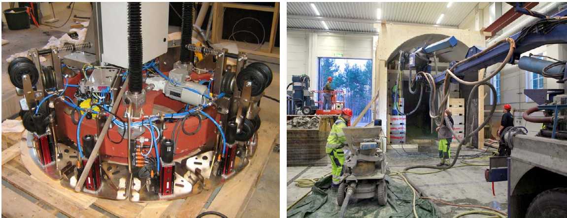
Figure 5-2. Left: Installation tool for the buffer. Right: Pellets installation test in backfill.
